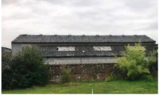
1.13 The front building in red facing brick and a cement sheet roof was constructed in
